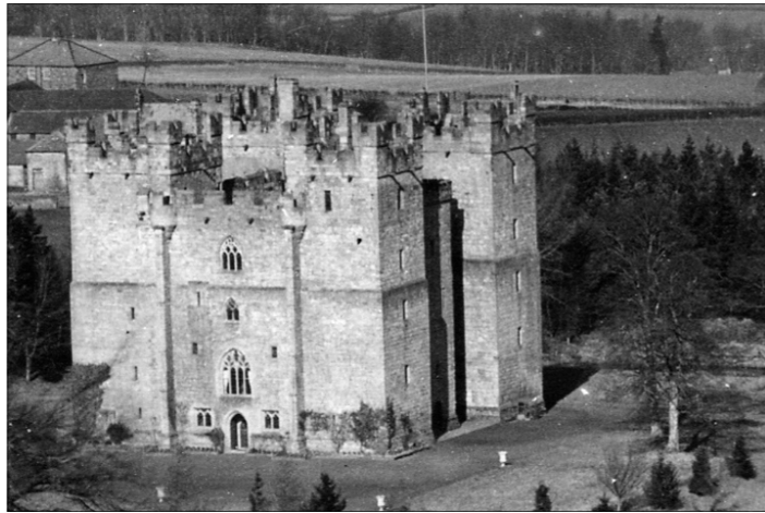
Langley Castle : the Bates' restoration completed with the rebuilding of the North-West 'Bell Tower' and the South-East 'Chapel Tower'
