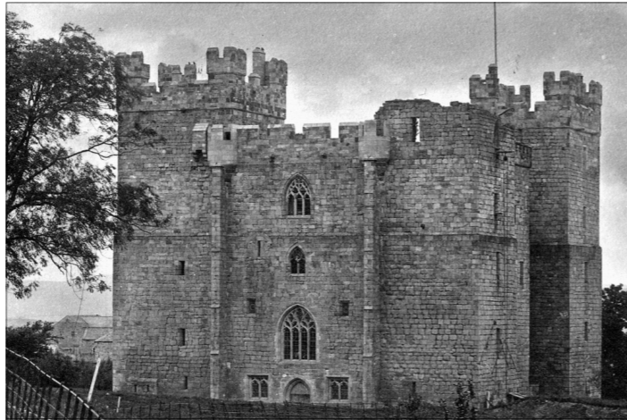
Langley Castle : two towers Restored
