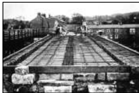
The surface of the old bridge is replaced : 1910
