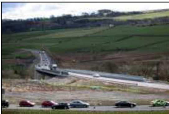
The west bound lane of the Haydon Bridge Bypass opens. 25-03-09 @ 11.30am
