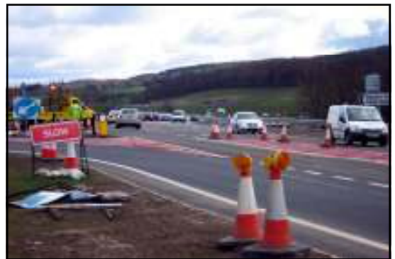
The east bound lane of the Haydon Bridge Bypass opens. 25-03-09 @ 11.37am
