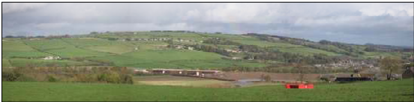
HAYDON BRIDGE BYPASS. 26th October 2008
